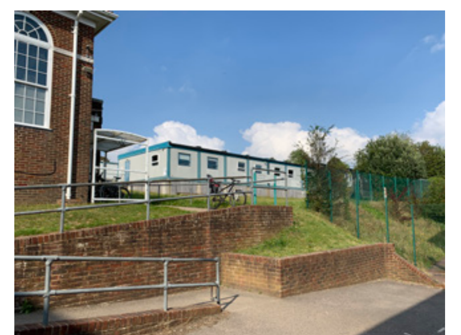
Temporary Classrooms view from Car Park
