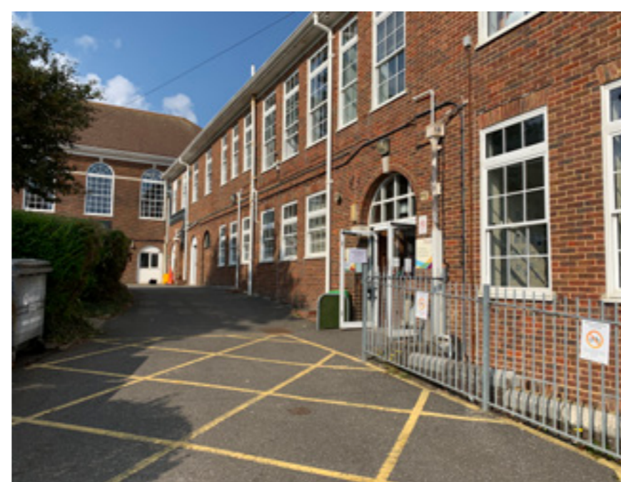
Main Building East Entrance
